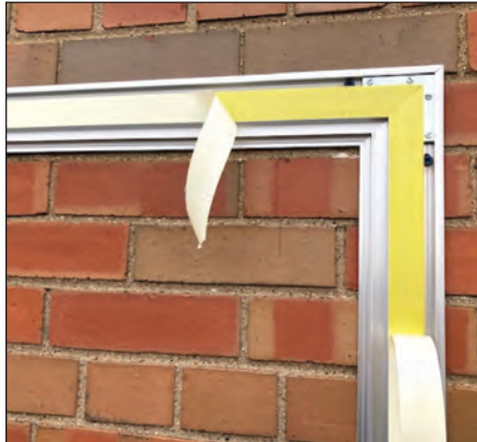
Remove masking. Tack down banner on left and right vertical BASE rails and pull tight.
