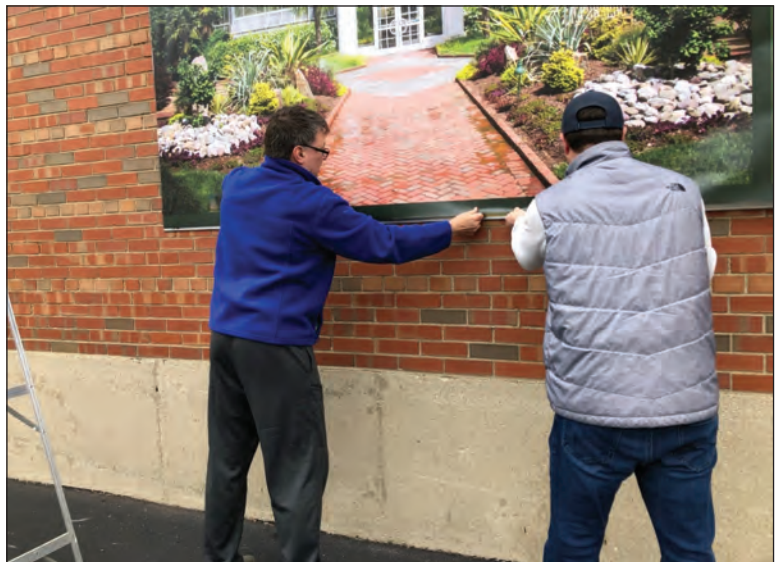
To achieve a wrinkle free banner, you must have the banner tacked to all 4 BASE rail sides in a smooth, tight, wrinkle free manner before putting the CAPS on. You can pull off the banner from the tacky tape and reposition as needed.
